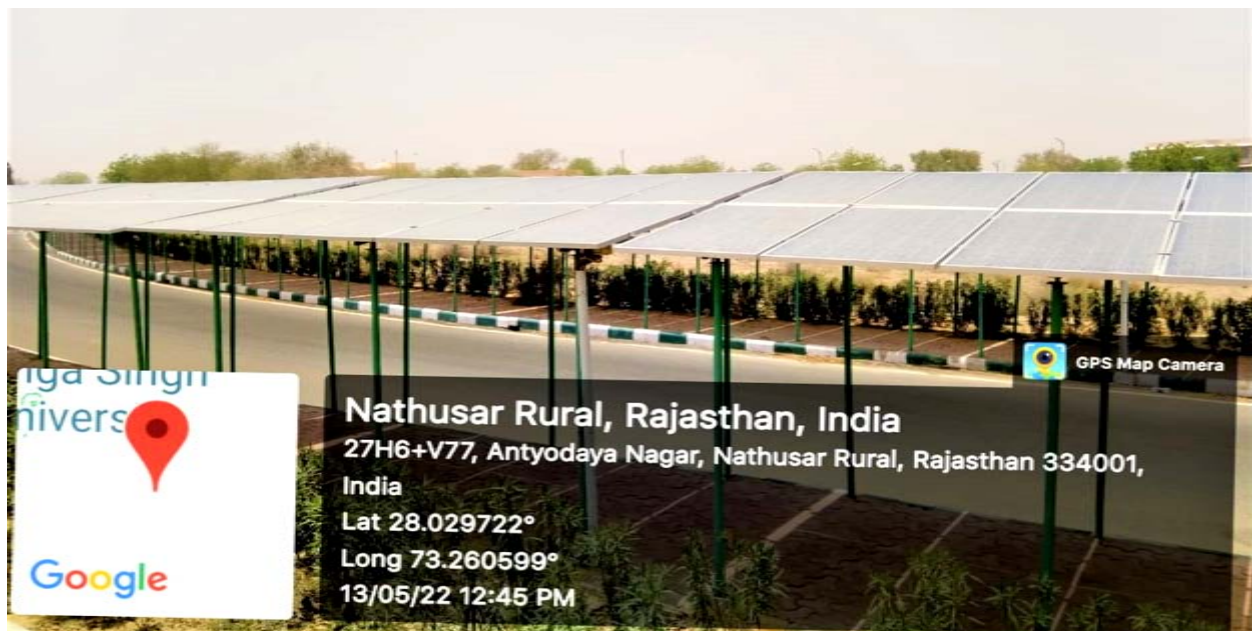
Installation of Solar Panels at MGSU
